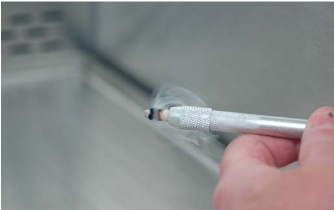
Airflow at sidewalls being pulled under work surface
